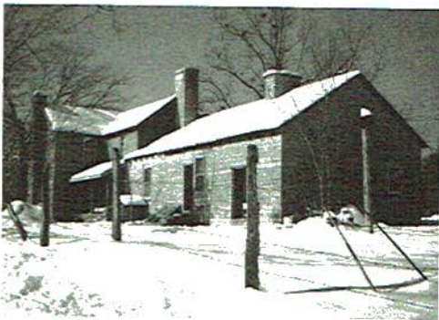
The house of Capt. James Doran in Doran's Cove. The front part has been added in later years. The back part stands today as it did then
