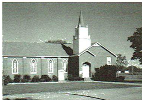
Section United Methodist Church
